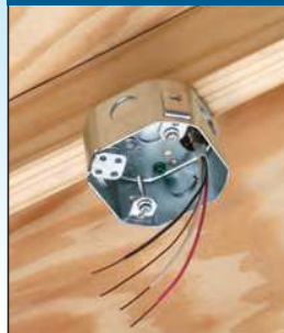
FBS415/FBS420 Mount UNDER Joist
